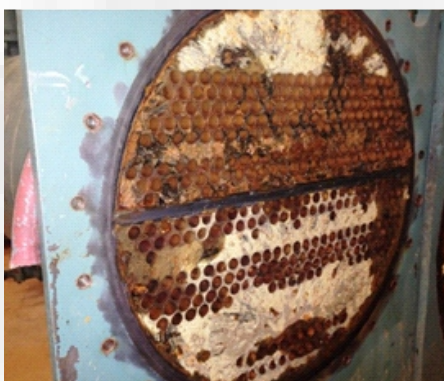
Heat Exchanger Repair & Protection
