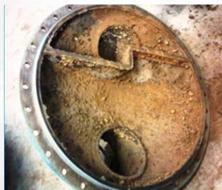
Heat Exchanger Repair & Protection
