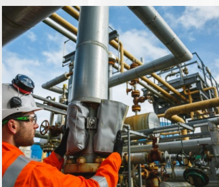
Heat Exchanger Repair & Protection
